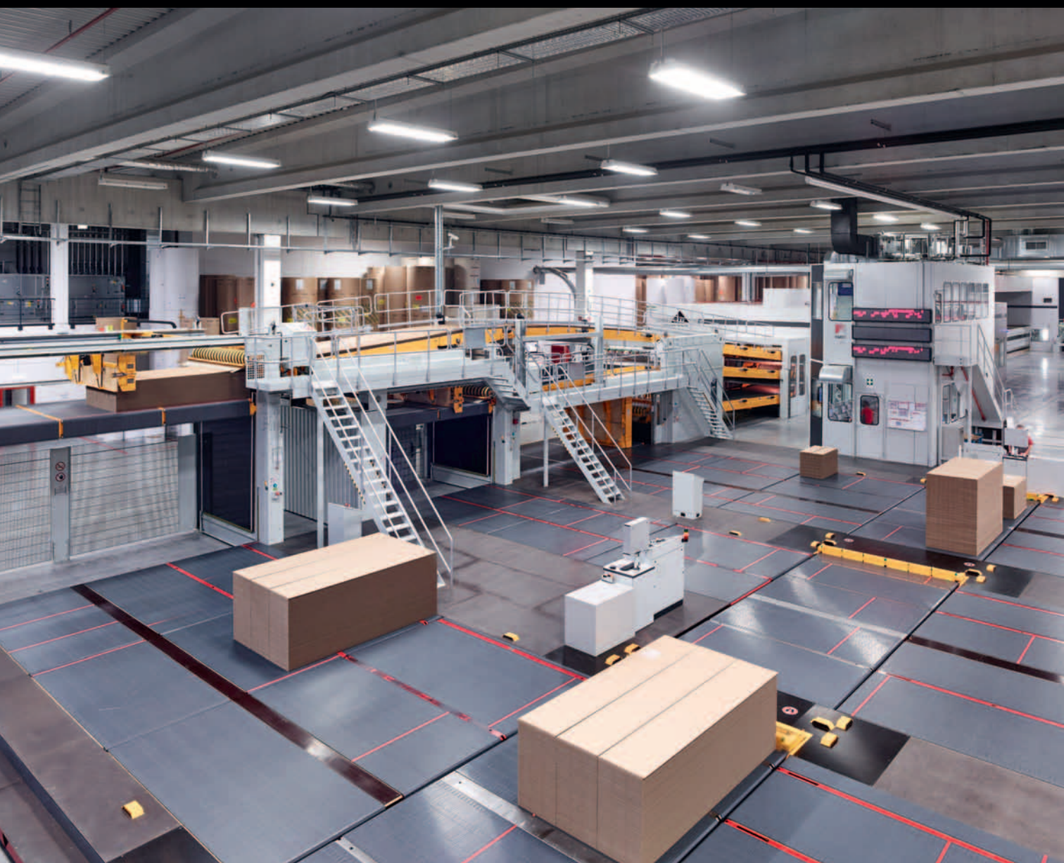
BHS Corrugated Sortieranlage
